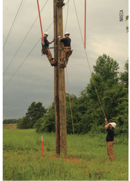
Four County EMC linemen replacing a pole for distribution line.
