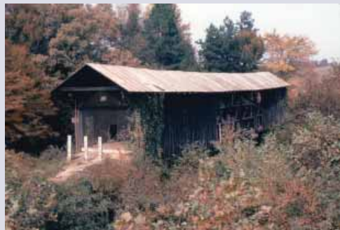
Eddie Hough made one of the last photos of Skeen's Mill Bridge, the state's oldest covered bridge, which spanned the Uwharrie River near Flint Hill northwest of Asheboro. It fell down in 1987.
