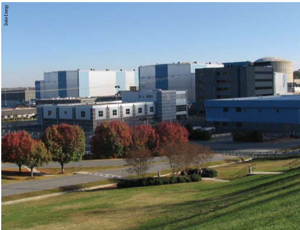
The Catawba Nuclear Station in York County, S.C., began commercial operation in the mid-1980s and recently was relicensed to operate through 2043. North Carolina’s Touchstone Energy cooperatives own 56.25 percent of one of the two Catawba generating units.
