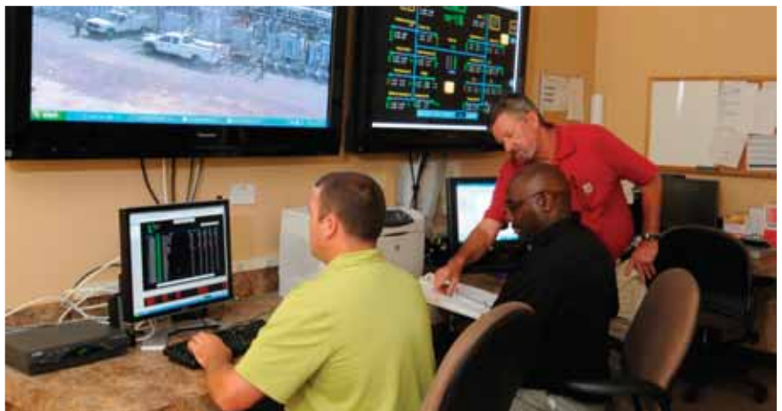
Reviewing plans for substation upgrades are (from left) Sandhills Utility Services engineering manager David Keith, CEO Jeffery Brown, and operations manager David Austin.
