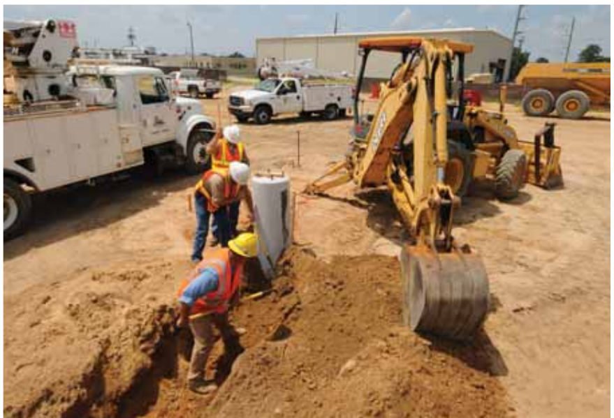
A construction crew installs concrete light bases.
