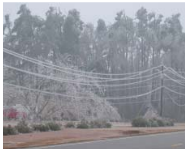
Ice coated power lines and trees in the Carvers Creek area of Bladen County, served by Four County EMC.
